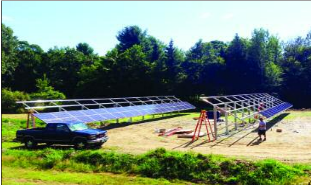
First two rows of racking being outfitted with panels.
