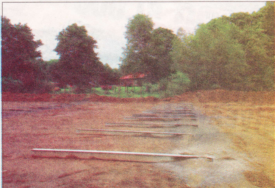
Solar racking sits in the ground shale from freshly drilled holes.
