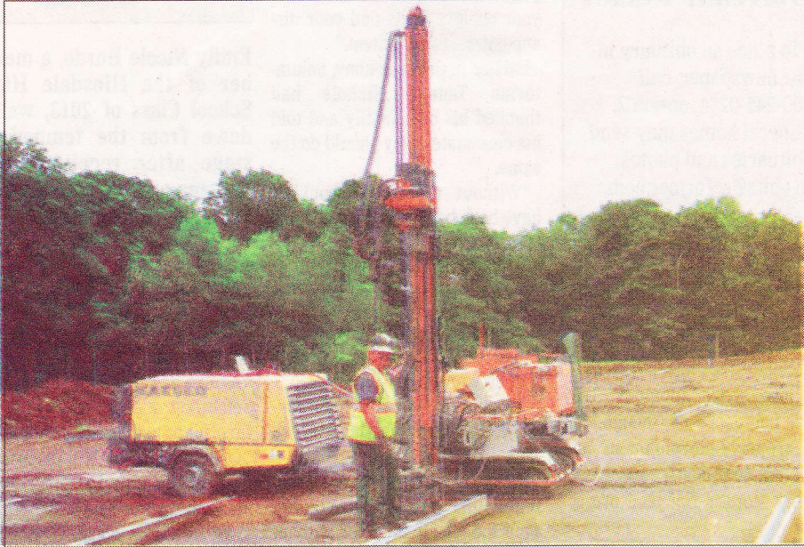
Drill operator Jeronimo Torres prepares to drill 4 feet into ledge.
